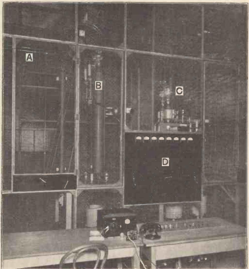
The last two stages of the W<sub>2</sub>XMN transmitter. A, input line from earlier stage. B, push-pull driver stage. C, push-pull output stage. D, meters for the two final stages; their needles remain quite stationary during operation.
