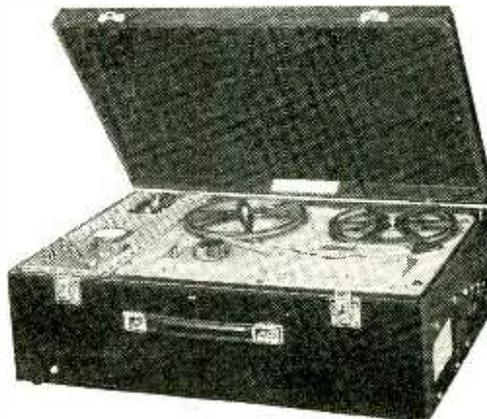
The amplifier, speaker and case, with detachable lid, measures 8½ in. x 22½ in. x 15¾ in. and weighs 31 lb. Price £49, to which cost of Tape Unit to your choice, must be added.
