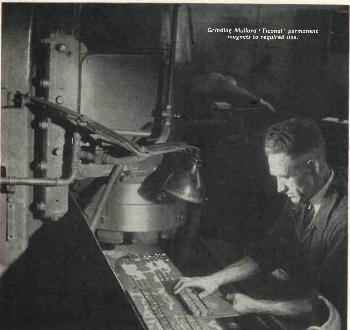
*Grinding Mullard 'Ticonal' permanent magnets to required size.*
