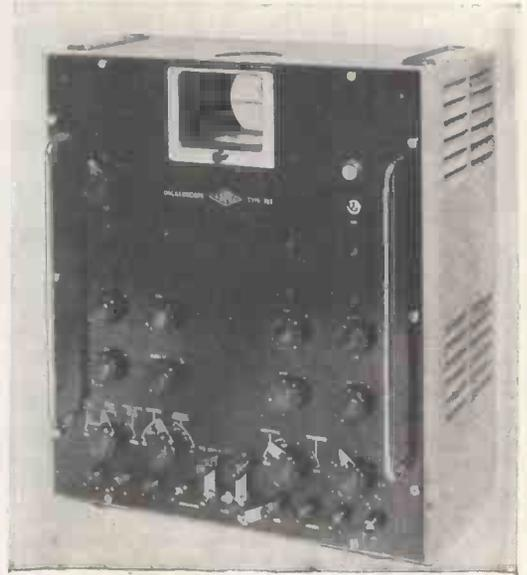
THE OSCILLOSCOPE CAMERA TYPE 758 is designed specifically for use with Airmec Oscilloscopes. It may be used for single shot photography or continuous recording, and a motor with variable speed gearing is included for the latter purpose. The cassettes will accommodate 100 feet of 35 mm. film or paper and a footage indicator shows the amount of film used.
