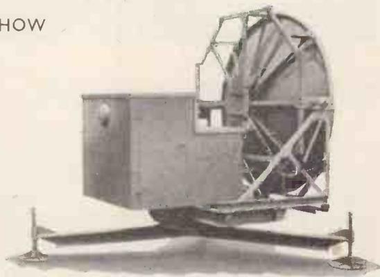
Decca "Wind-Finding" radar; the operators sit in the enclosed cabin behind the aerial "dish."
