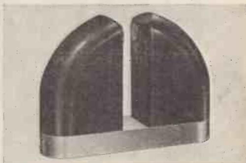
Another example, illustrated above, shows a fully protected 'horn' shaped magnet which gives a magnetic field in the gap of 5500 oersts and weighs only 14 lb. A particular feature of this magnet is that it is specially designed to give an accurate and stable performance under the worst possible condition of usage. It can be brought into contact with iron and steel and other magnets and still remain within the manufacturer's specification and retain its magnetic calibration.
