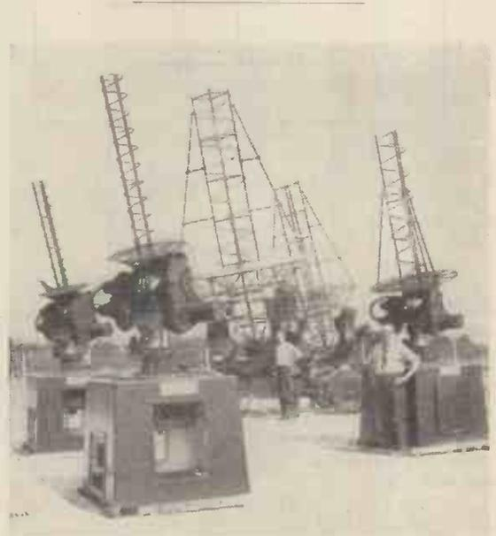
FRAME-GRID AERIALS?—These five helical aerials have been designed by Cossor Radar & Electronics and are for use by the War Office at the Guided Weapons Trials Establishment on the coast of Anglesey. They will operate in the frequency range 100—400Mc/s employing circular polarization and will be for telemetering missiles.
