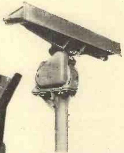
Above: The end-fed slotted waveguide aerial of lightweight construction gives a beam width of  $1.9^\circ$  with a 4ft horizontal aperture.
