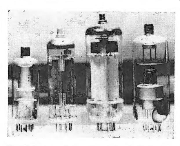
Mullards first range of valves designed specially for time base and e.h.t. circuits of colour television receivers. From left to right: E.H.T. rectifier GY 501, booster diode PY 500, line output pentode PL 505 and shunt stabilizer triode PD 500.
