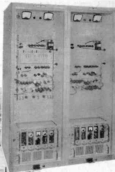
▲ A Pye microwave (6-8 Gc/s) transmitter and receiver as supplied for the Tower.
