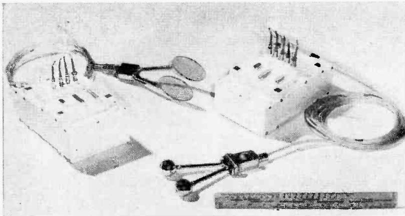
Fig. 2. Instrumentation for measuring electron temperature (spherical probes) and density (Birmingham University). To ensure good electrical connections between screened sections of the two modules, each part which is machined from Duralumin is gold plated to a thickness of 0.0001 in.
