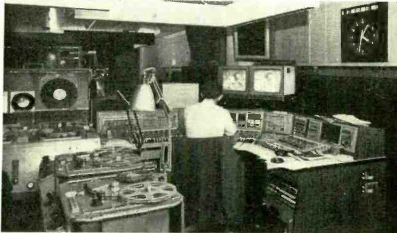
Sound controller's position with tape and disc backing facilities, in the sound control room associated with one of the two colour studios.
