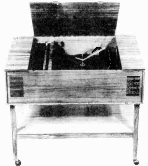
*Dynatron model HFC4 "Geneva" transistor c. radiogram with decoder fitted. Long- and medium-wave and v.h.f. coverage, 20W power output. Bass reflex speaker enclosures. Record changer with diamond stylus. Price: £111 8s 8d plus stand.*
