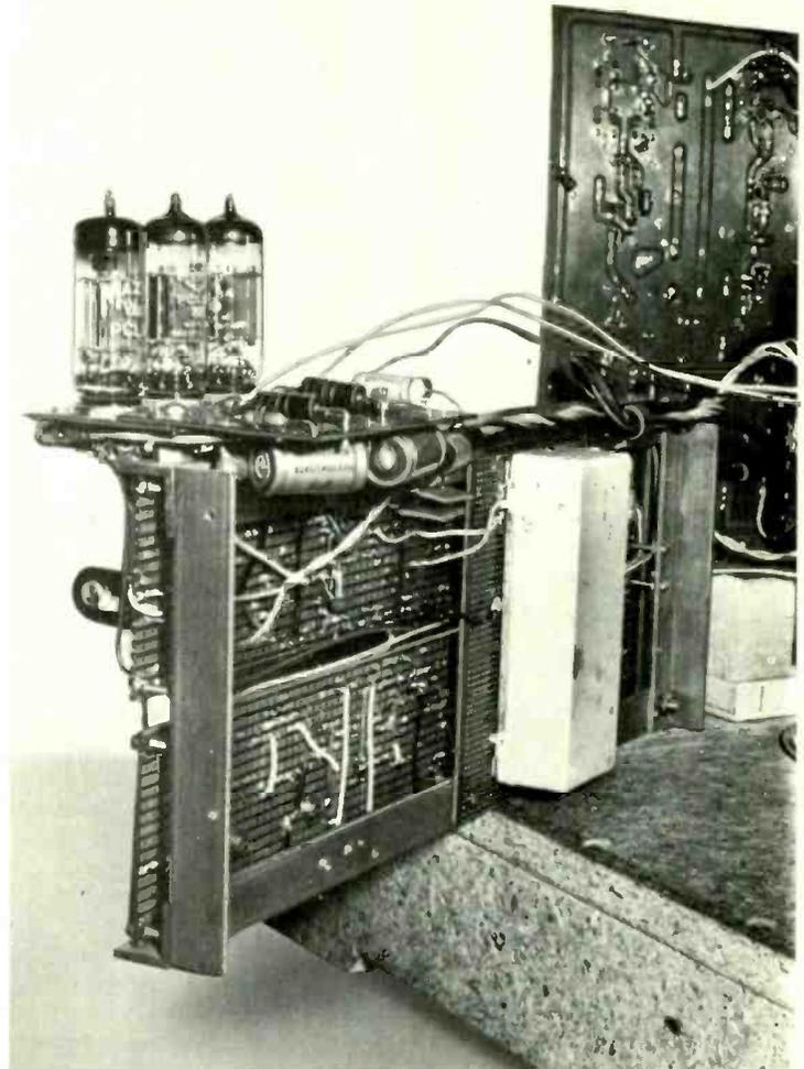
The decoder section opened out and showing the PAL delay line.
