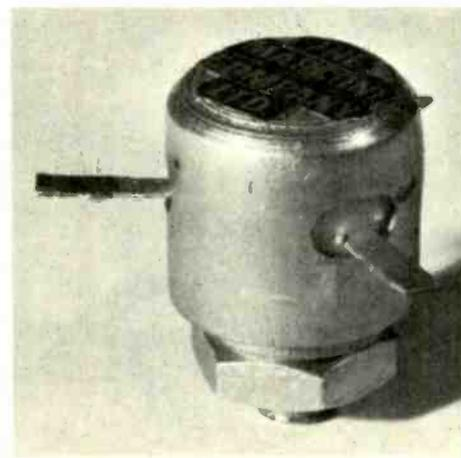
printed circuit and micro-strip work and is magnetically screened to minimize the effects of stray external fields. Its rugged construction enables it to operate in severe environmental conditions. Three types are available. Type F1024-04 has a range of 200-400MHz, F1024-05 a range of 250-500MHz, and F1024-06 a range of 300-600MHz. Instantaneous bandwidth is 3% typical for 20dB isolation. Insertion loss is less than 1dB. Power handling capacity is 10W. The Marconi Co. Ltd, Chelmsford, Essex.
