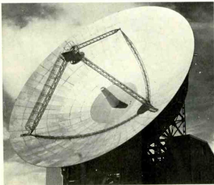
*The Cassegrain aerial system of the new Goonhilly satellite communications station is a 90-ft dish some 350ft above sea level, and has the advantage that when a satellite is on a nearly stationary orbit tracking can be effected by movement of the sub-reflector and without having to move the main dish.*
