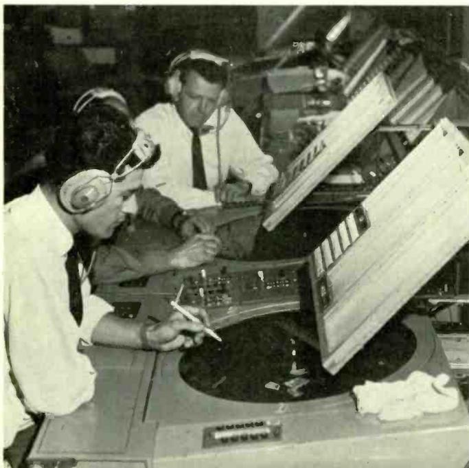
*Controllers at work during a Mediator simulation. Recently the equipment was used to determine which was the best site for London's third airport from an air traffic control point-of-view; Foulness came out tops.*
