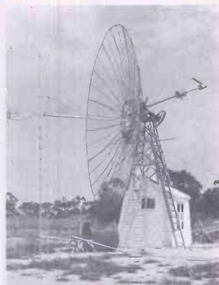
This 28ft diameter dish was made by the Australian amateur VK3ATN for his moon-bounce experiments. The reflector uses half-inch mesh. Gain is 38dB at 1296MHz and 28dB at 432MHz. The photo was taken by L. A. Moxon (G6XN) during a recent visit.
