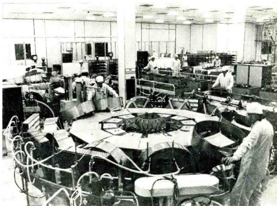
*Flow-coat mill of Mullard's £10M television picture tube plant at Durham. The equipment in this section of the mill applies a layer of phosphor dots on the face of the tube. The dots provide the blue content of the picture. Similar equipment is used to apply the red and green phosphor dots.*
