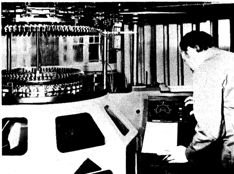
Vernon H. Cooper Ltd's new yarn speed monitor can be used in conjunction with all types of knitting machines, both circular and flat and having varied rates of feed. The monitor incorporates EMI's electronic fabric control system.
