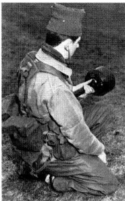
Fig. 11. Small portable radar torch (SPRAT) in use. Photograph by courtesy of the Royal Radar Establishment who developed the unit.
