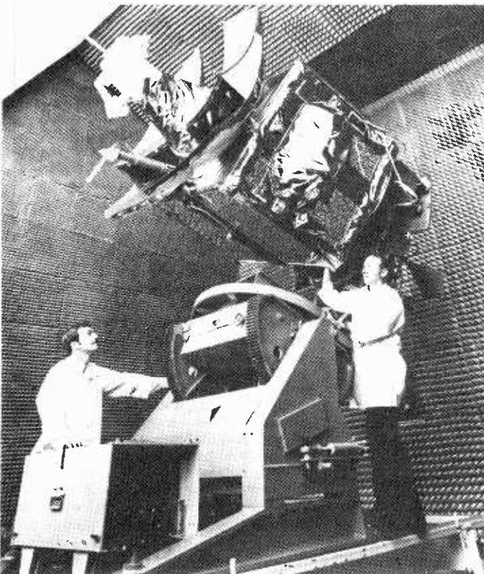
*Satcom II during tests of the antenna system at RCA's Astro-Electronics Division, Princeton, New Jersey. The domestic communications satellite has recently joined Satcom I in orbit. It is capable of providing a communications service to 50 North American states.*
