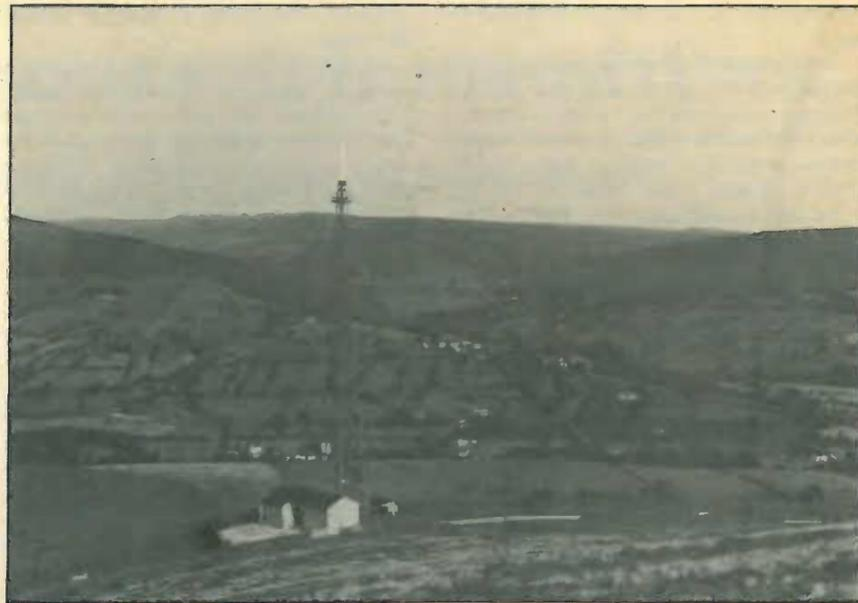
Shatton Edge. The 'slimline' tower was originally developed for use in the Peak District National Park. The 'trough' receiving aeriels are just above the special stone building. The cantilevered cylinder contains a 'cardioid' transmitting aerial.
