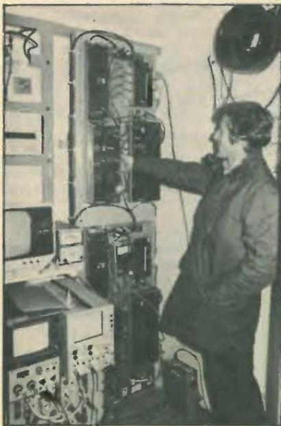
Inside Hedleyhope. Gordon Bowhay, of the BBC's transmitter capital projects department, is putting the finishing touches to his 'Blue Streak' installation. The instruments at bottom left are test gear, not station equipment.
