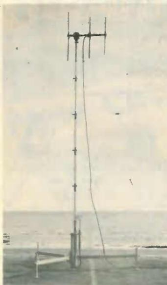
Telescopic air operated Clark Mast Type QT4m/HP mounted on portable tripod.
