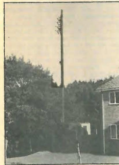
Tötley Rise, Sheffield. One of the BBC's tiny, unobtrusive installations with wooden pole, log-periodic aerials and prefabricated building.
