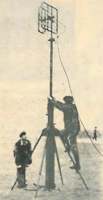
Mobile air-operated 21-metre telescopic trailer mast. Horizontally stowed for transit, raised to vertical position for extension.
