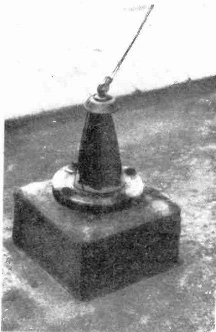
Fig. 3. Feed through insulator of emergency aerial.
