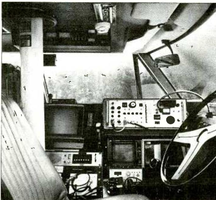
Receiving, demodulating and measuring equipment inside a BBC survey vehicle.
