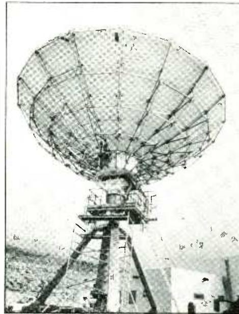
One of two 13m C-band antennae being installed by Marconi at Whiehill, Oxon as part of an Inmarsat earth station for Mercury Communications.
