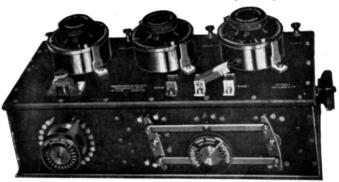
The' Marconi Multiple Tuner for adjusting to the various Wave Lengths.
