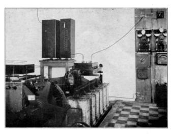
The Rolary Spark Gap, Oscillating Transformer, and Inductances.
