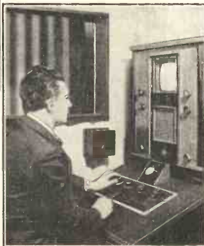
A glimpse inside the German television station at Berlin from which ultra-short-wave high-definition transmissions are sent. The top photograph illustrates a portion of the transmitting equipment, while that on the right shows the control apparatus.
