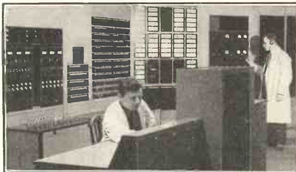
This photograph is typical of German efficiency, and was taken in the Berlin control room. The main control desk is seen in the foreground, while a special indicator, which shows which studios are in use, is visible in the background.
