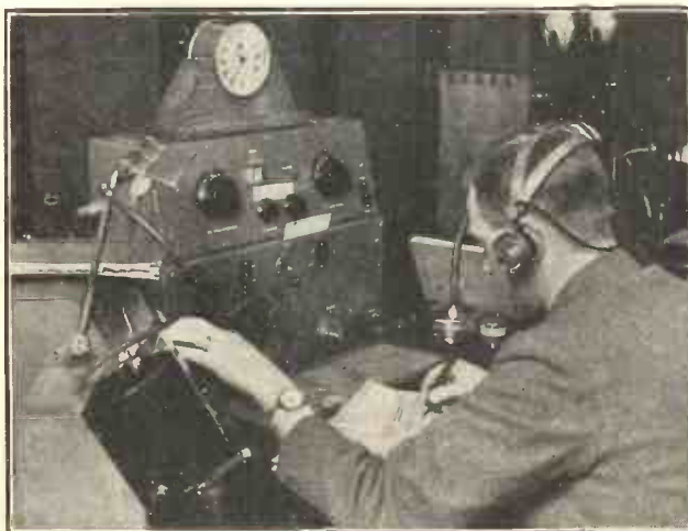
Courtesy of the Postmaster-General A typical scene at a G.P.O. coastal radio station. A radiogram from a ship at sea is being received.
