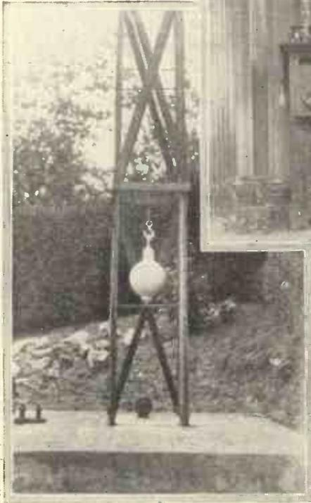
A very high-class amateur station, showing the receiver fitted into an antique sideboard, and the 55 ft. lattice mast. Note the weight for keeping the aerial under constant tension.
