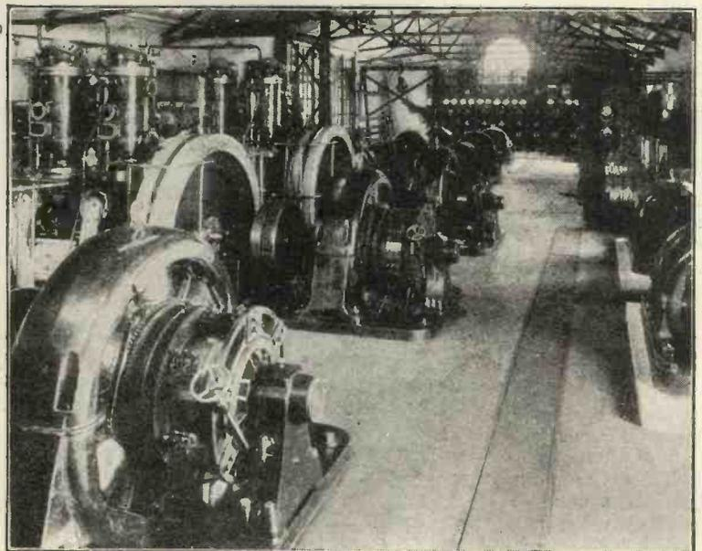
*View of the central power house, showing direct-current generator and motor alternators.*
