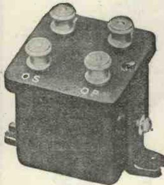
Fullers United Electric Co.'s inter-valve transformer.
