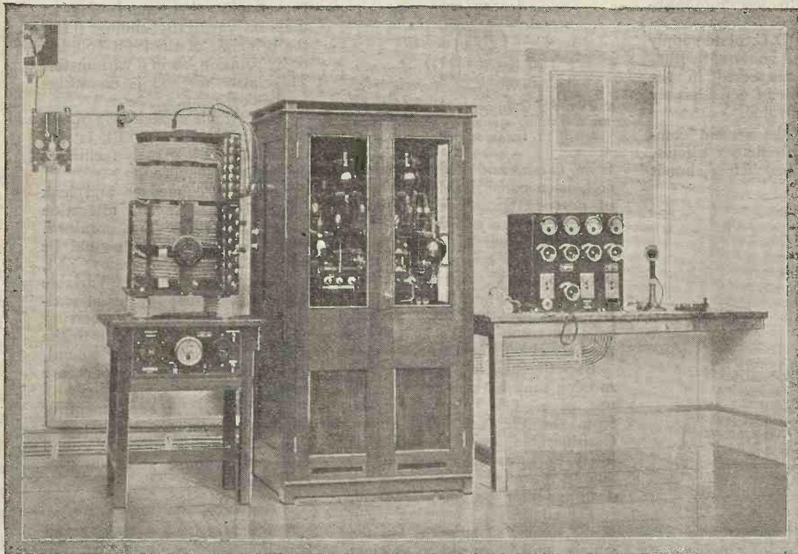
The compactness of a modern valve transmitting station is well illustrated in the above photograph showing a combined wireless telegraph and telephone station. Only the tuning and transmitting controls are exposed. (Photo. Marconi's Wireless Telegraph Co., Ltd.)
