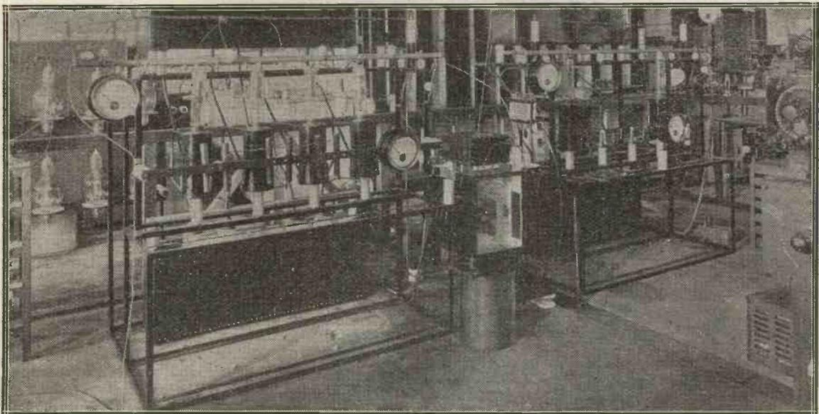
Water-cooled valves in use at the high-power broadcasting station at Chelmsford (5XX).
