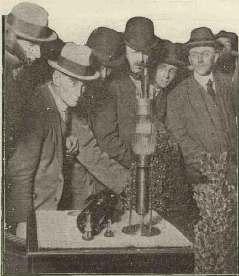
*A contrast in valves which may be seen at the Exhibition, the large one being a ten kw. water-cooled transmitting valve.*
