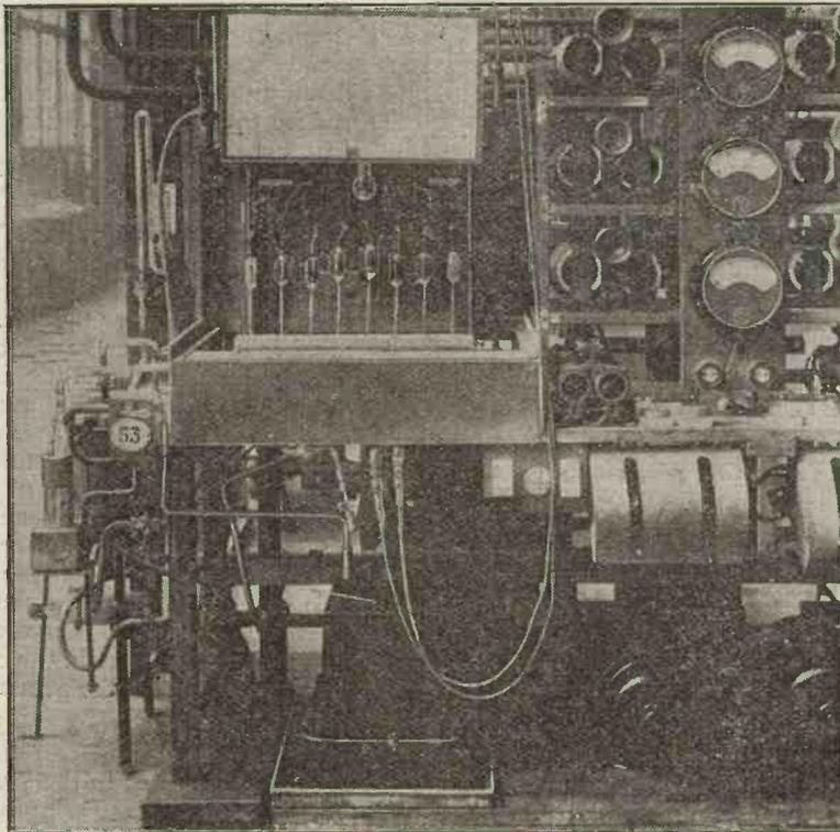
*Pump tables with eddy current heating equipment for fine filament valves.*
