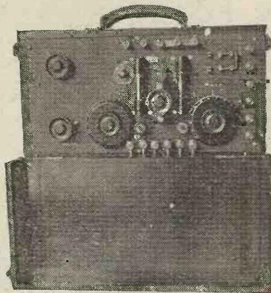
A portable two-valve receiver made by a "Wireless Weekly" reader.
