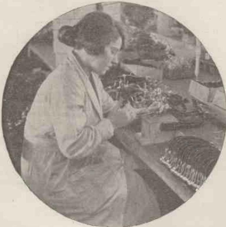
*Our photograph shows one of the operations in the manufacture of the B.T.H. headphones. The end of the stirrup is being bent to prevent the slides from coming off.*
