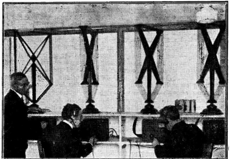
A loud speaker in each apartment and four plug sockets in the walls simplify radio for tenants in one of New York's newest block of flats. A central station on the top floor boasts four radio sets and an operator. Four stations are tuned in, and every tenant has the choice of plugging in on one of them. Our photograph shows two of the sets being tuned.
