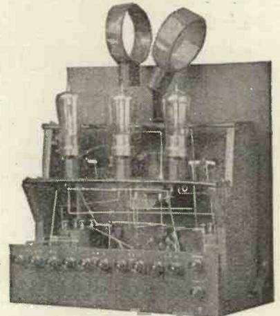
Mr. Scarborough's three-valve receiver seen behind the panel.
