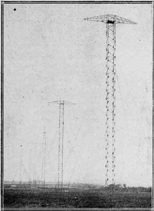
*Six of the ten masts to be used for supporting the aerial system at the Beam station at Bodmin, Cornwall, now being constructed by the Marconi Co. for communication with Canada and South Africa.*
