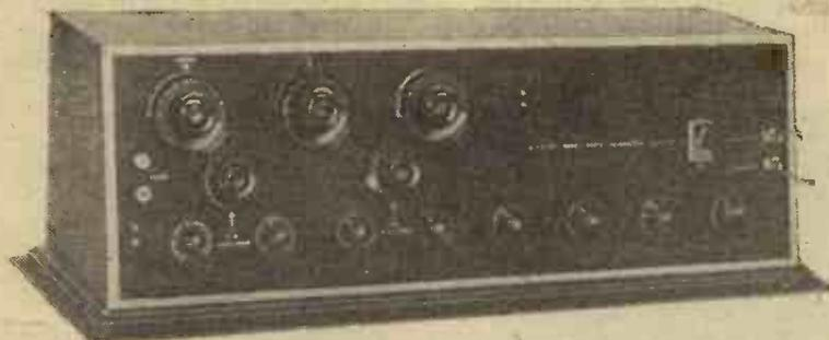
An eight-valve superheterodyne designed by Mr. Scott-Taggart, incorporating a stage of tuned H.F. in front of the first detector.
