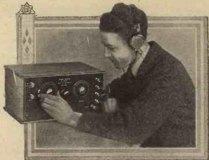
**T**HE choice of suitable dials for the tuning controls of a receiver has been the subject of a previous article in this series. The comfort of the operator is an important factor in fine tuning, for which reason special dials are often an advantage. A further trouble which may be encountered, especially at the higher frequencies, is that of hand-capacity.
