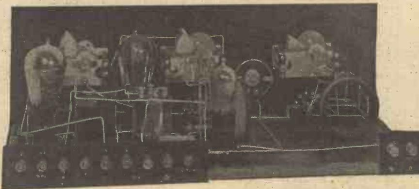
The special disposition of the coils should be particularly noted and copied. This is an important point when the wave-trap must be placed in fairly close proximity to the receiving circuits.
