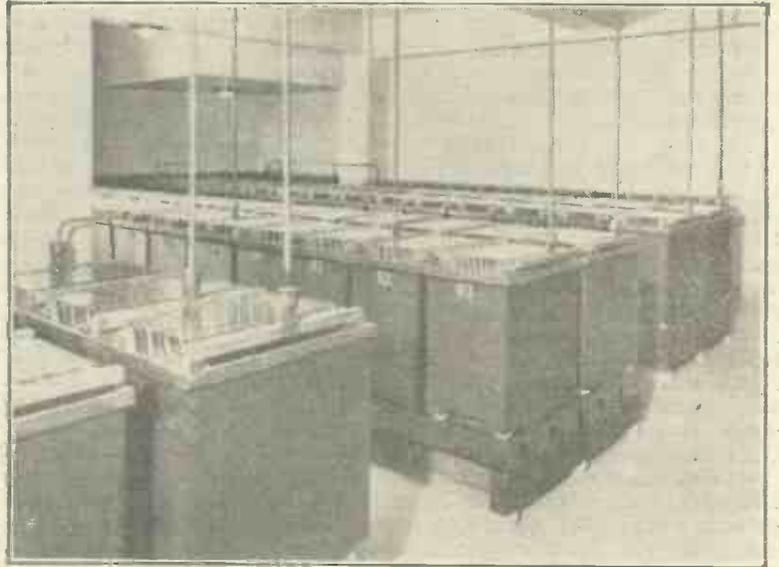
Main storage battery—240 volts, 1,000 ampère-hours—for emergency lighting supply
