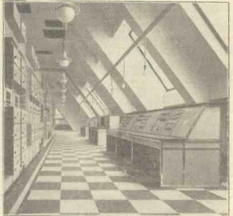
Fig. 2—Transmission Control Positions and Amplifiers in Control Room
